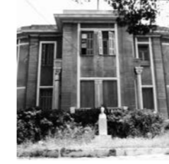
BUILDING RESTORATION P. Faliro, Athens, Greece Project Phase > Detailed Design Total Area > 520,00 m 2 Owner > General Airforce Headquarters Client > ERGOKAT S.A.
