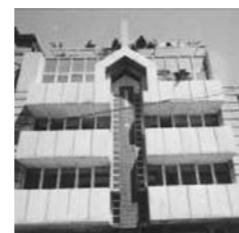
OFFICE BUILDING Kyrilou Loukareos st. Lycabettus, Athens, Greece Project Phase > All Phases Total Area > 1,200 m 2 Client > Th. & K. Boukas
