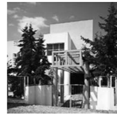
STATE PRE-SCHOOL DAY CENTER II Paleo Faliro, Greece Project Phase > Complete Design Total Area > 1,700 m 2 Owner > Ministry of Health and Welfare Client > I.&Th. Papaioannou, IASON TECHNICAL S.A.
