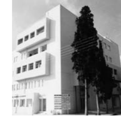
OUTPATIENT CLINIC SOCIAL INSURANCE TRUST FUND Piraeus, Greece Project Phase > Complete Design Total Area > 2,005 m 2 Owner > I.K.A. Technical Department Client > MELKA Ltd
