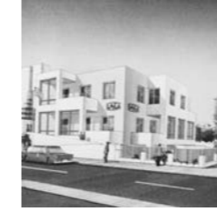
OAED PROFESSIONAL TRAINING SCHOOL Athens, Greece Project Phase > Detailed Design Total Area > 1,780 m 2 Owner > OAED Client > AVAX S.A.
