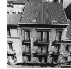
RESTORATION OF AGEA ETHNIKI BUILDING Athens, Greece Project Phase > Complete Design Total Area > 1,500 m 2 Client > Ethniki Insurance Company In Collaboration With > D. Vlahopoulos 50%
