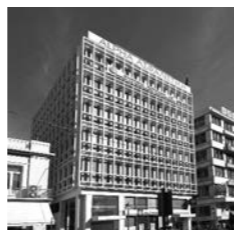
ALPHA BANK OFFICE BUILDING Omonias - Fotila St, Kavala, Greece Project Phase > Preliminary Design - Detailed Design - Working Drawings - Building Permits Total Area > 3,411m 2 Client > ALPHA BANK S.A.
