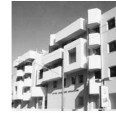
OUTPATIENT CLINIC SOCIAL INSURANCE TRUST FUND Kolokyntou, Athens, Greece Project Phase > Complete Design Total Area > 1,884 m 2 Owner > I.K.A. Technical Department Client > MELKA Ltd
