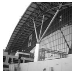
GALATSI SHOPPING CENTRE Athens, Greece Project Phase > Working Drawings Total Area > 84,000 m 2 Client > Park Avenue Development of Shopping Centers in Collaboration with > ARCHICON S.A. 50%
