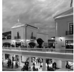
McARTHURGLEN ATHENS DESIGNER OUTLET MALL Spata, Attica, Greece Project Phase > All Phases Total Area > 65,000 m 2 Client > McARTHUR GLEN HELLAS Ltd in Collaboration with > ARCHICON Ltd. 50%
