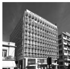
ALPHA BANK OFFICE BUILDING Omonias - Fotila St., Kavala, Greece
